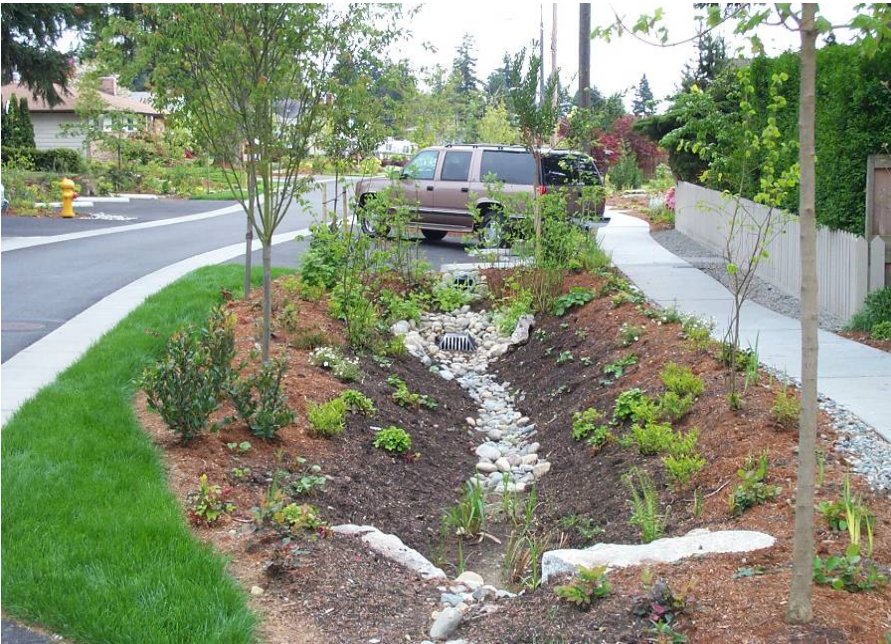
A bio-swale in place of curb and gutters and storm sewers.
