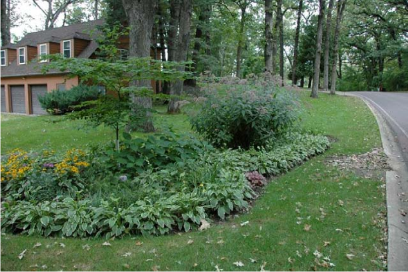
A rain garden in Okoboji takes street runoff through a curb cut. Runoff that used to go directly into West Okoboji Lake now gets infiltrated, cleaned, and slowly released – as groundwater flow to the lake.
