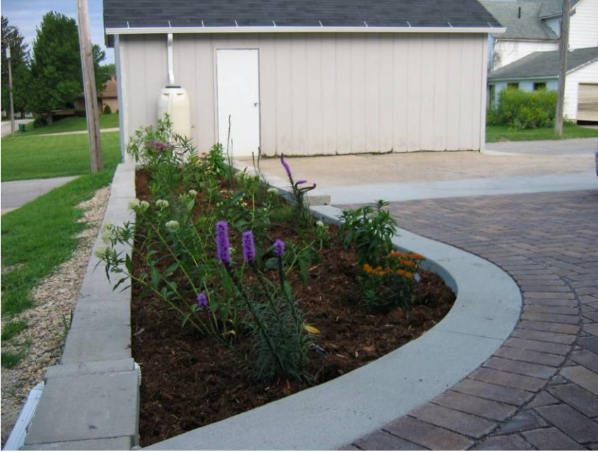
A rain garden in the back of Woodard Insurance - a downtown business in West Union. Roof runoff enters the rain garden through the downspout (seen in the lower left corner of the picture). Permeable pavers are to the right of the rain garden and a rain barrel takes roof runoff from the garage in the background – making this a three practice project.
