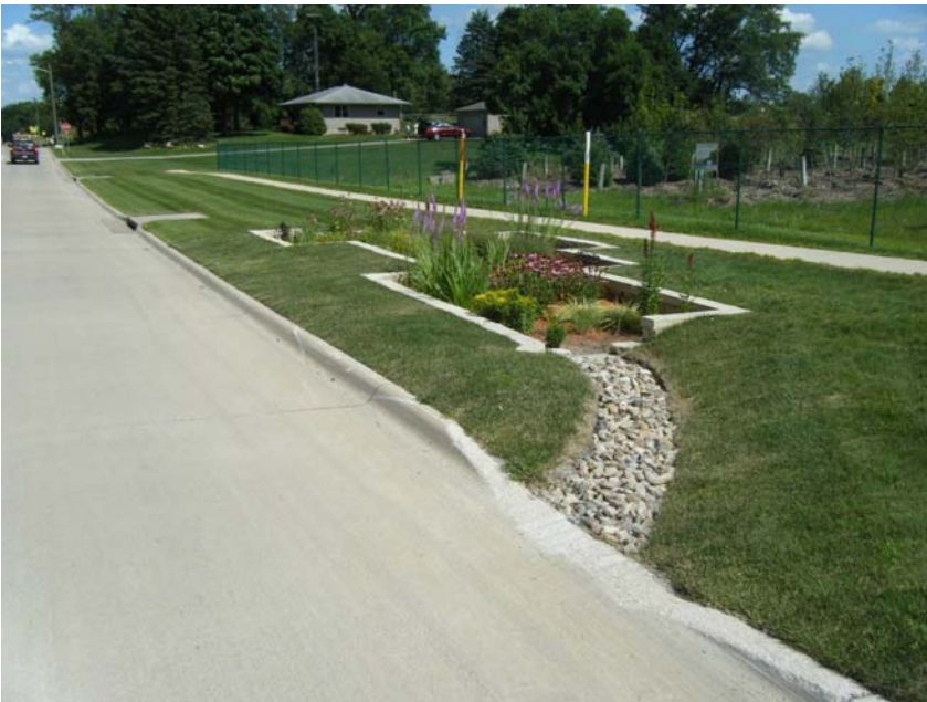
A rain garden in Coralville takes street runoff through a curb cut. Note the storm sewer intake in the background. Most of the time dirty runoff won't get to the storm sewer.
